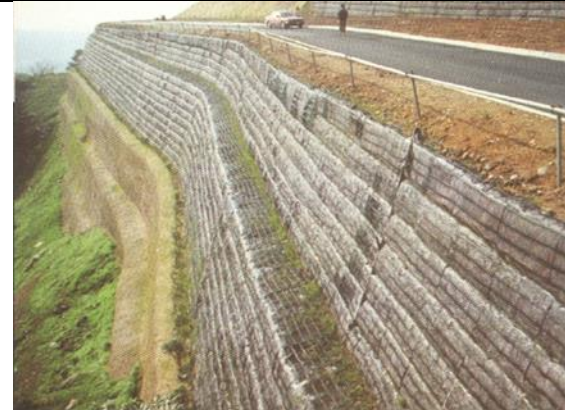
Vegetation develops quickly on slopes constructed with soil-filled bags (Taiwan). Such structures can be designed to withstand seismic loadings.
